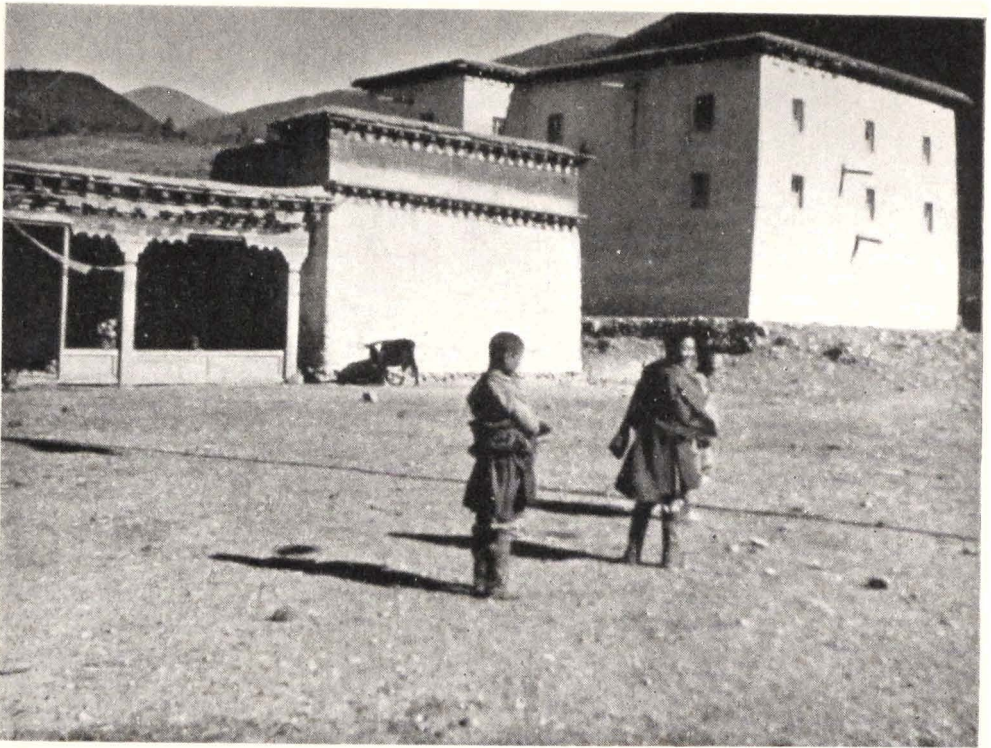
3. Pangdatshang's house in Bo, with a family temple on the extreme left. The wooden channels projecting from the wall of the house on the right are part of the primitive plumbing system and carry away the waste water
